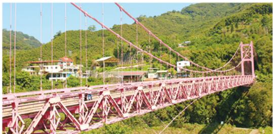
The 150 m long Fuxing Bridge is the first grand-scale, cable-stayed suspension bridge in Taiwan. Spanning high above the beautiful Dahan Creek, it integrates both transportation and observatory functions with its footpath and balcony.
